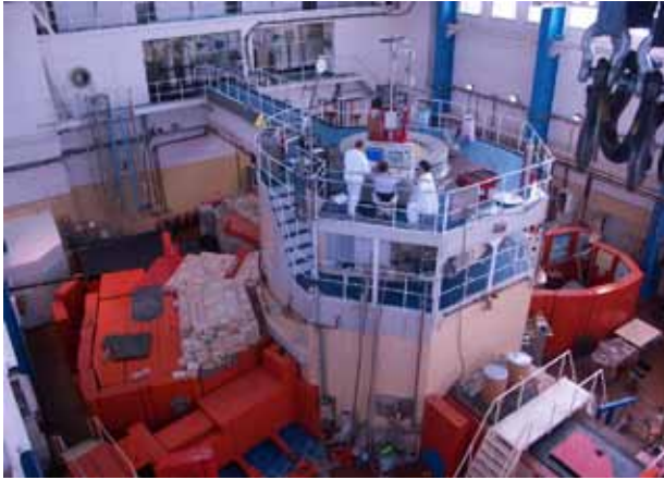
Panorama view of Reactor Hall
