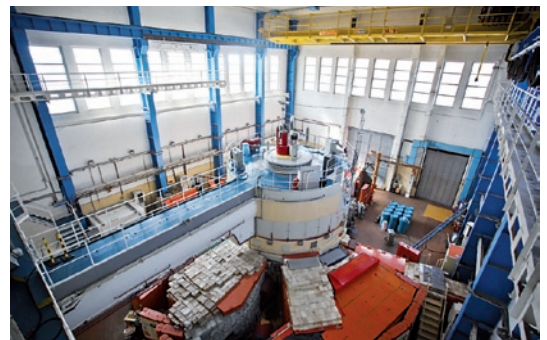
▲ Panorama view of the Reactor Hall
